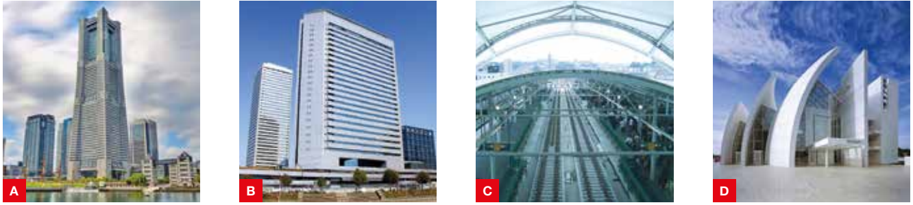
Şekil.7-Applications of self-cleaning exterior building materials. Top left to right: a) MM Towers in Yokohama coated with self-cleaning tiles, b) Matsushita Denso building covered with self-cleaning glass. Bottom left to right: c) Self-cleaning roof of a train station in Motosumiyoshi d) dives in Misericordia Church, Rome, Italy (10).
